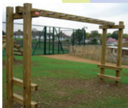
Horizontal Ladder [TT15] SS: 32m 2 /FFH 1.8m
